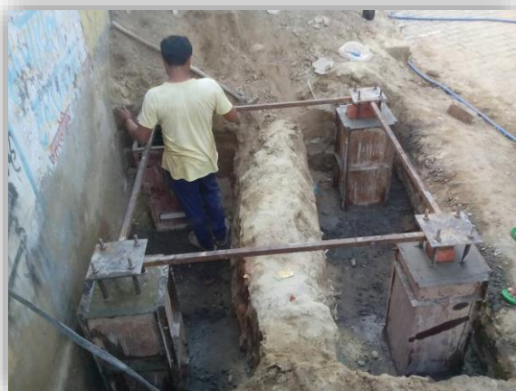
Structure Foundation work
