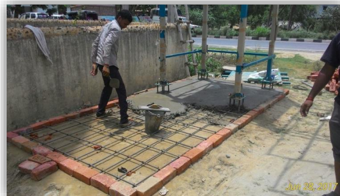
Structure Platform work
